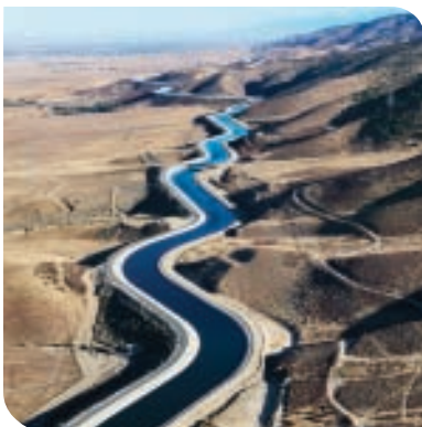
State Water Project
