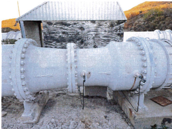
Looking downstream at new ultrasonic meter installation & vent pipe
