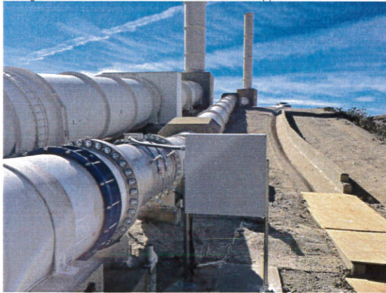
Looking downstream at new ultrasonic meter installation & vent pipe
