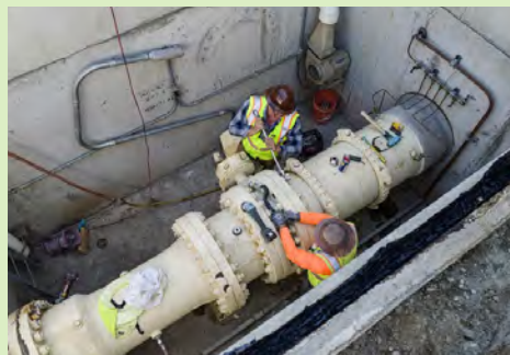
The Hydro 24-inch Butterfly Valve Replacement Project.
