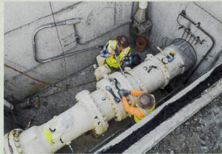
The Hydro 24-inch Butterfly Valve Replacement Project.
