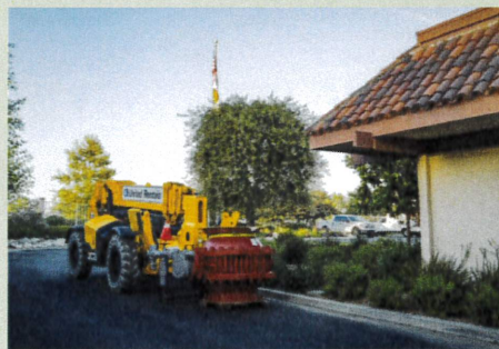
The San Gabriel Flow Control Structure 30-inch Ball Valve Replacement Project.
