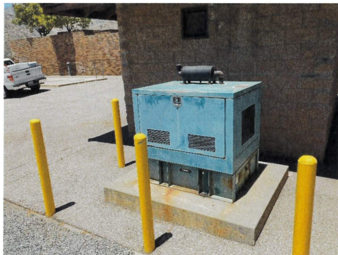
Figure 7.2 – Existing Generator to be Replaced.
