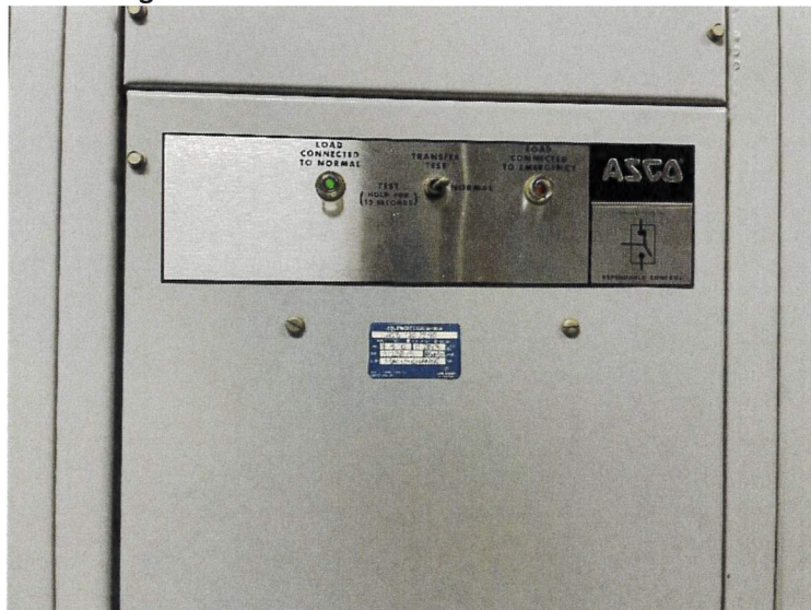
Figure 5.2 – Automatic Transfer Switch Section
