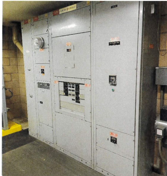
Figure 5.2 – Automatic Transfer Switch Section
