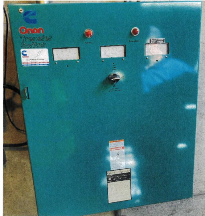
Figure 3.4 – Existing Automatic Transfer Switch to be Replaced
