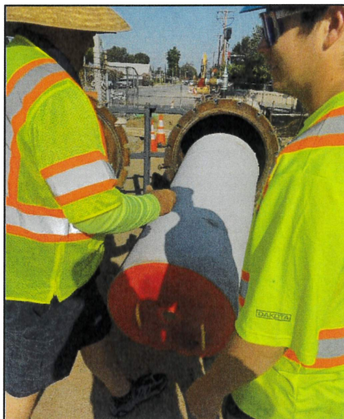
Figure 6. Technicians insert the cleaning pig into the launch barrel.
