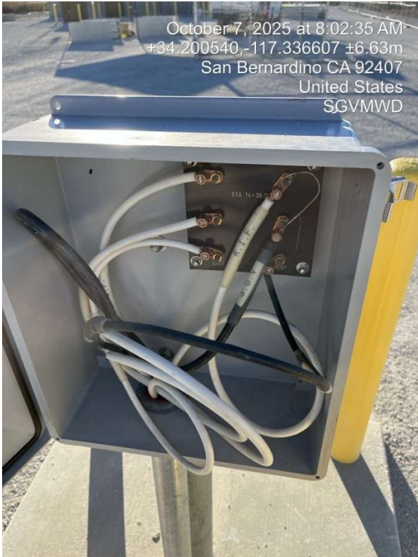
Schedule VI – Sta. 1999+60 Bonding Test Station
