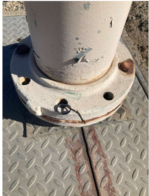
Schedule VI – Sta. 1896+85 ETS Test Station
